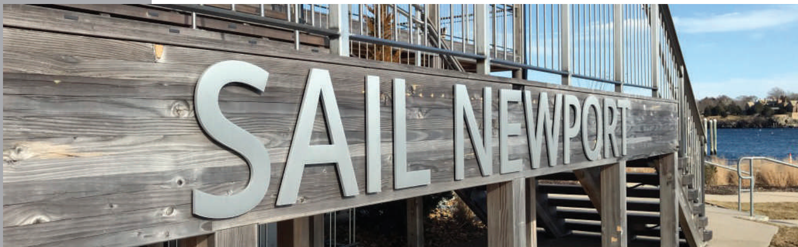
1/4" THICK STAINLESS STEEL LETTERS STUD MOUNTED TO WOOD
