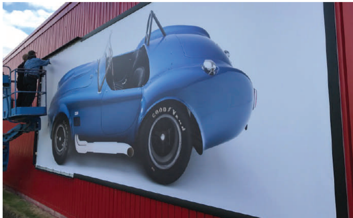
14 OZ. 10FT. X 30FT. BANNER MOUNTED IN CUSTOM INTERCHANGEABLE ALUMINUM FRAME
