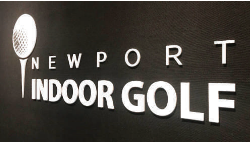
CNC 1/2" THICK FOAMCORE VELCRO MOUNTED TO CARPET WALL
