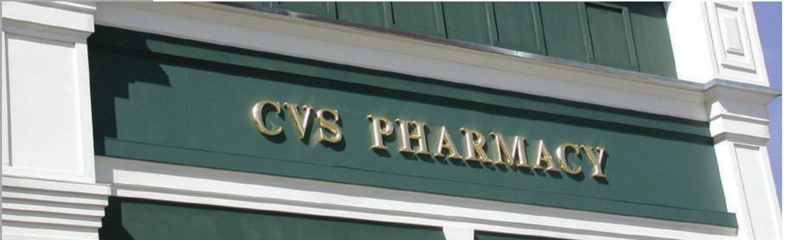
MOLDED ROUND FACE LETTERS GILDED WITH 23 CARAT GOLD LEAF, STUD MOUNTED TO WOODEN FACADE
